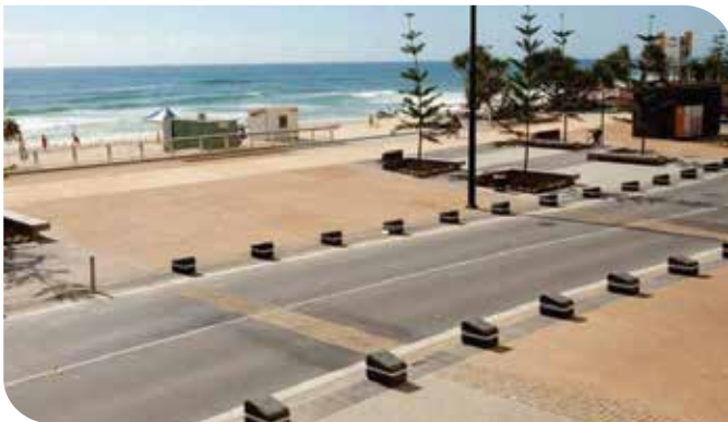
Pathway completed with CCS Kalgoorlie
